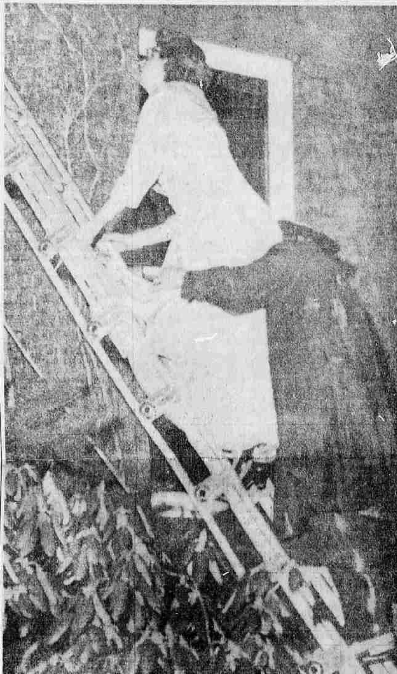
ESCAPES FLAMES - Mrs. Nelson Rockefeller, wife of the governor of New York, is shown being helped down a ladder by a fireman as fire broke out in the Executive Mansion in Albany, N. Y., early today. Rockefeller said damage to the house and valuable art collection would run about half a million dollars. (UPI Telephoto)
