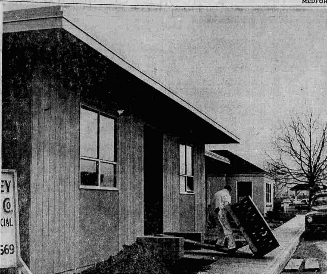
MOVING DAY —Equipment is taken into the new building on Highway 99, which houses the Oregon state police here and the area office of the public utilities commissioner.
