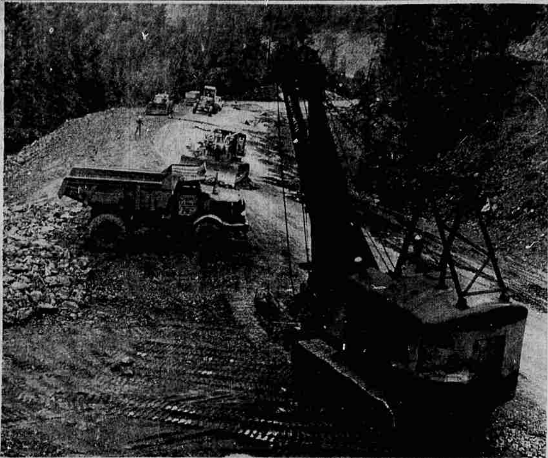
PROGRESSING —Work is progressing on straightening and widening sections of Highway 62 between Shady Cove and Prospect. The area pictured is about 10 miles south of Prospect. Construction was started late last summer. Bulldozers and scrapers are shown removing large rocks from the road surface. Most blasting work has been completed on the sections. Paving will be completed later this year.
