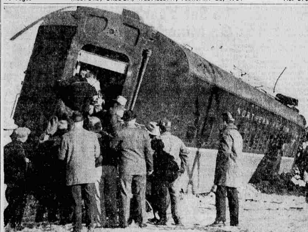
WRECK VICTIM ASSISTED—One of the 43 passengers injured in the derailment of the Northern Pacific Main-streeter passenger train near Buffalo, N.D., is assisted from
