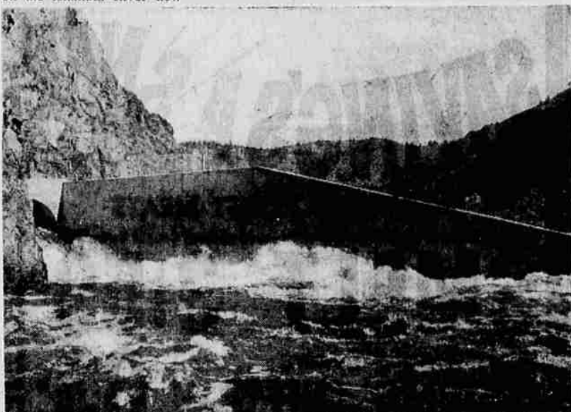
SPILLWAY — The Klamath River foams through the spillway opening on the left as the water is diverted around the main site to allow for construction of the Iron Gate dam. The truck in the center of the picture is working on the coffer dam at the tunnel entrance. The main dam will be built 173 feet high between the tunnel opening and the coffer dam.
