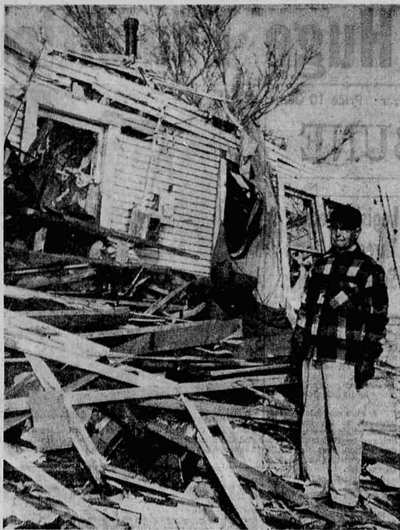
HOME DESTROYED—H. H. Amberg stands amid the rubble of his home, splintered by a million damage near Konawa, Okla. Amberg also lost a house in a fire a few years ago. (UPI Telephoto)
