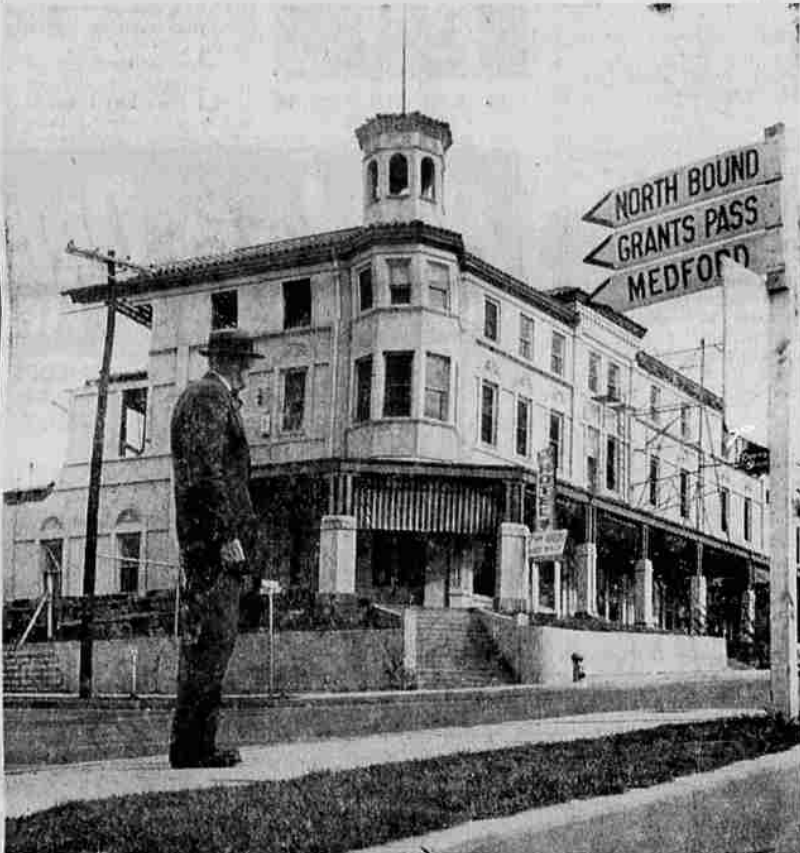
MANY MEMORIES — Clarence Lane, 90, of Ashland, looks on as wrecking crews busy about demolishing the Ashland hotel. The 72-year-old hotel holds many memories for Lane. He has raced, marched
