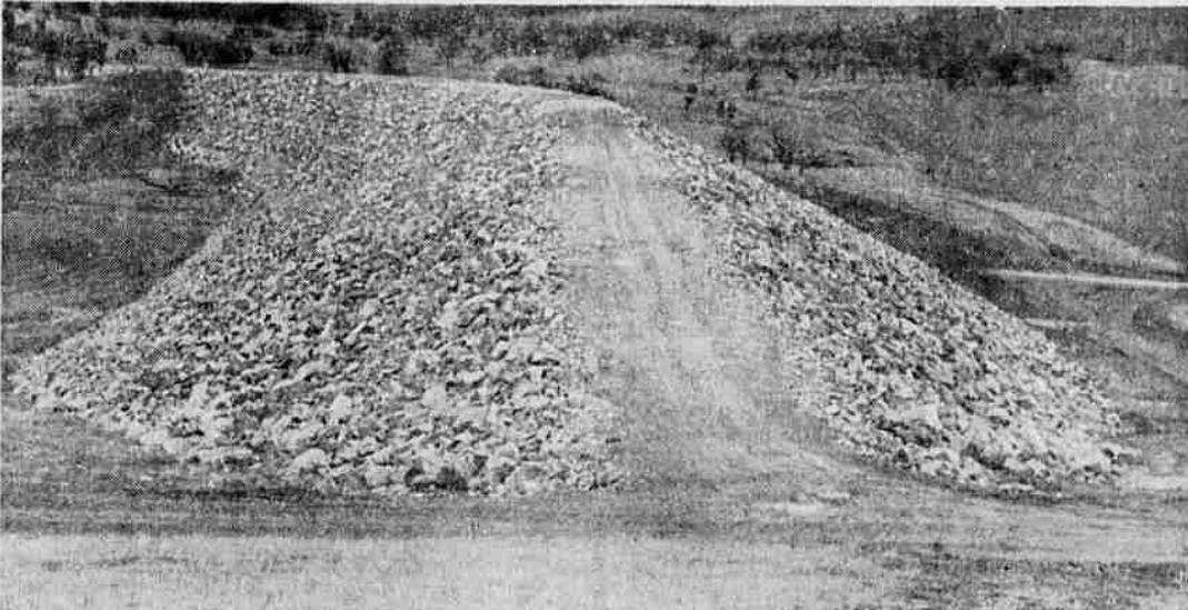
The concrete outflow works, connecting with a tunnel under hill abutment at left, can be seen dimly behind trees in lower left of picture.
