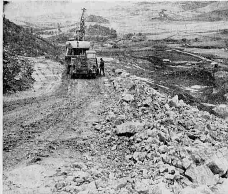
ROCK SURFACING — The outer surface of the dam, shown above, is nearing completion, with a heavy coating of rocks and boulders. Equipment on access road at left, located below the crest of the dam, is finishing the job, which is expected to be completed within next few weeks. Much of the material for the dam was taken from the borrow pit seen far below; the rest of it was obtained from nearby clay-type areas.
