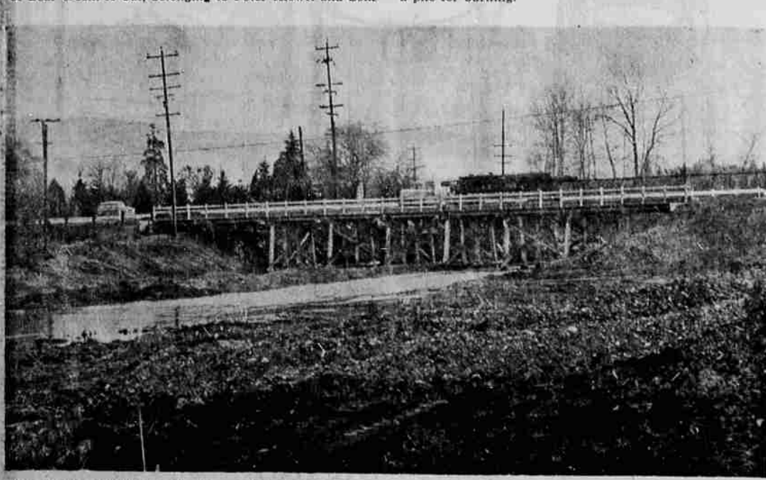
TEMPORARY DETOUR —Traffic on Crater Lake highway is being routed around the freeway construction by a detour bridge, pictured above. This detour, and another one
