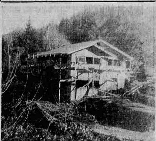
DISTRICT OFFICE—Construction is progressing on this new building which will be the Cow Creek district office of the Umpqua National Forest. The building is located on the bank of the Umpqua river near Tiller. Conference, engineering, drafting and sales rooms will be included in the new office.
