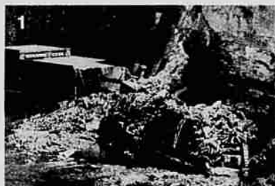
Niagara landslides crippled power plant.
