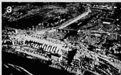
A new power project solves both problems.
