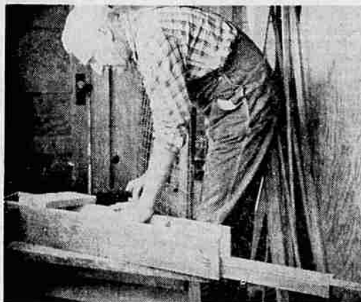
CARPENTRY WORK—Blindness hasn't stopped "Dad" Hanscom from leading an active life. He has been working on remodeling a house recently. He has done all carpentry work, plumbing and window installations. Hanscom says he considers blindness more of a nuisance than a handicap.
