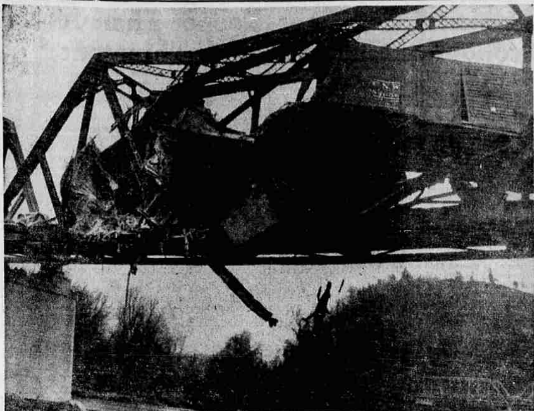
FREIGHT CARS DERAILED —Twenty one cars of a Frisco freight train were derailed on a bridge spanning the Gasconade river near Arlington, Mo. One person suffered injuries and a search was under way in the twisted wreck-
