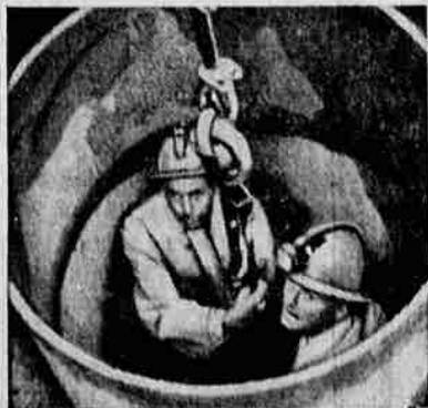
Only link to surface was pipe 42" wide, 40 stories deep. Lifty equipment was dismantled, lowered and reassembled on the cavern floor.
