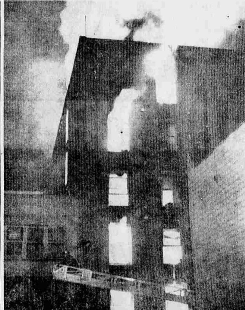
GENERAL ALARM FIRE - Flames shoot through the Thomas hotel in San Francisco in a general alarm fire that gutted the hotel, killed 18 persons, and injured at least 30 others. Note the fireman, bottom left, as he prepares to be taken up to evacuate possible survivors. (UPI Telephoto)
