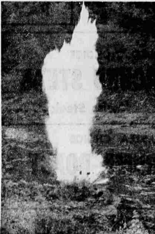
DEEPEN CHANNEL —A deeper channel is blasted through the rocks at Rainie Falls on the Rogue river downstream from Galice to improve fish passage.
