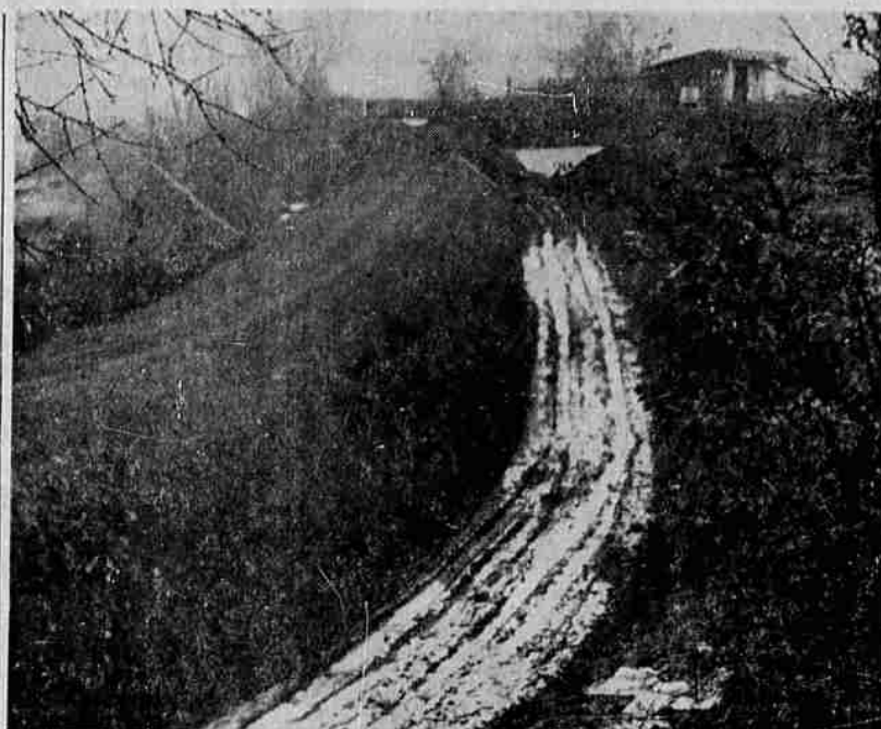
TALENT LATERAL —This shows the Talent lateral extending 20 miles on the west side of the valley. This picture was taken just off the old Phoenix-Talent highway. The project is under contract to Pacific
