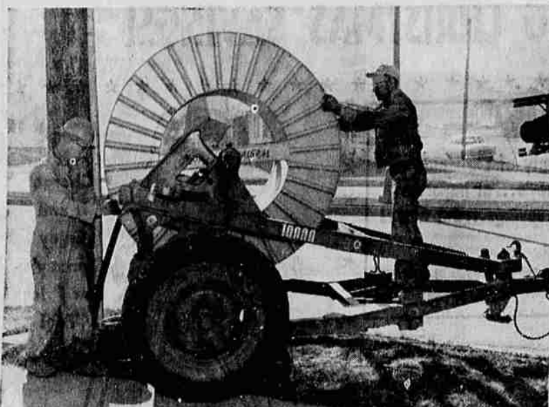
INSTALL CABLE - Bill Johnson, left, and Charles (Stan) Ludwig, construction line-men, are shown placing part of the three miles of underground cable for the new dial system in Ashland. The cable ranges in size from 900 to 2,100 pairs of wire. (Knackstedt Photo)
