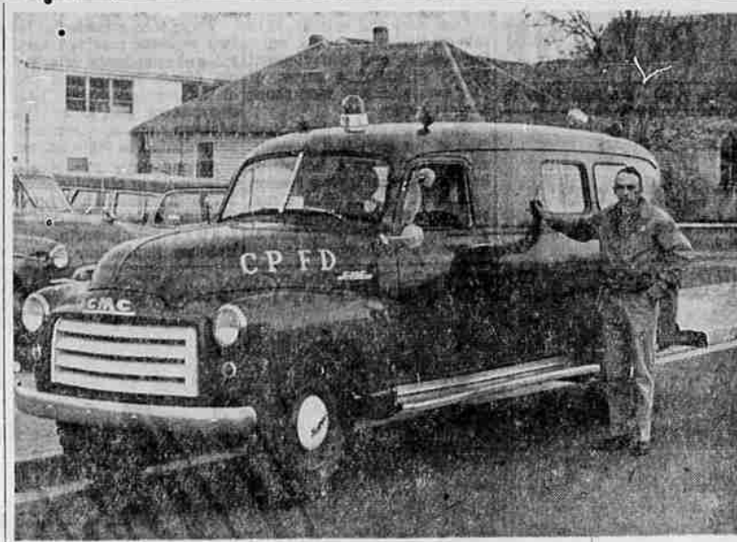
EMERGENCY RESCUE UNIT —The Central Point Volunteer fire department is finishing work on their new emergency rescue unit. The unit is available for use by all Rogue valley areas. Donald Milligan, fire chief, is pictured with the unit. Milligan and the 20 volunteer firemen have installed all equipment. A resuscitator, portable generator and underwater diving lung are included in special emergency devices.
