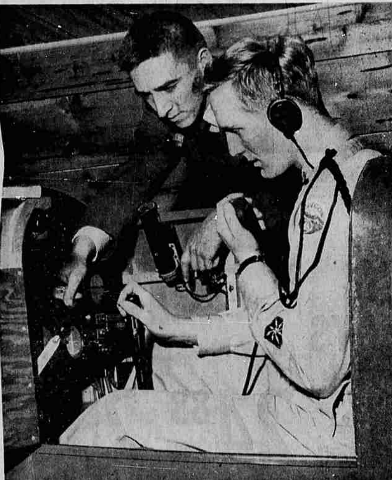
LINK TRAINER —CAP cadets and senior members get valuable experience by using this device known as a Link Trainer. The trainer is a model of an airplane cockpit, complete with instrument panel. Here Cadet Lt. Don Huntmann, cadet commander of the Medford squadron, is in the cockpit of the trainer. Lt. Bill Florey, senior training officer, is giving instruction.
