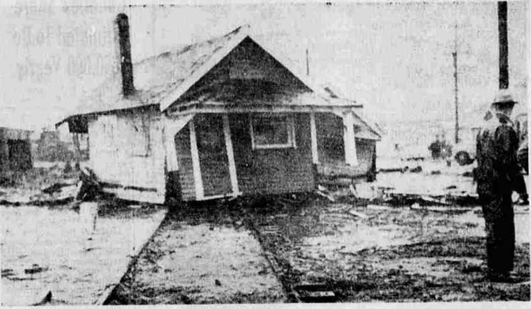
ROCKAWAY BATTERED —Residents of Rockaway, on the Oregon coast, estimate damage from a freak wave which struck in the early hours Wednesday to be close to $100,000. It was the second such wave within a month. The house shown in the picture was moved across the railroad tracks by the first wave. The owners had the home moved back to its original position only to have Wednesday's wave send it across the tracks. (UPI Telephoto)
