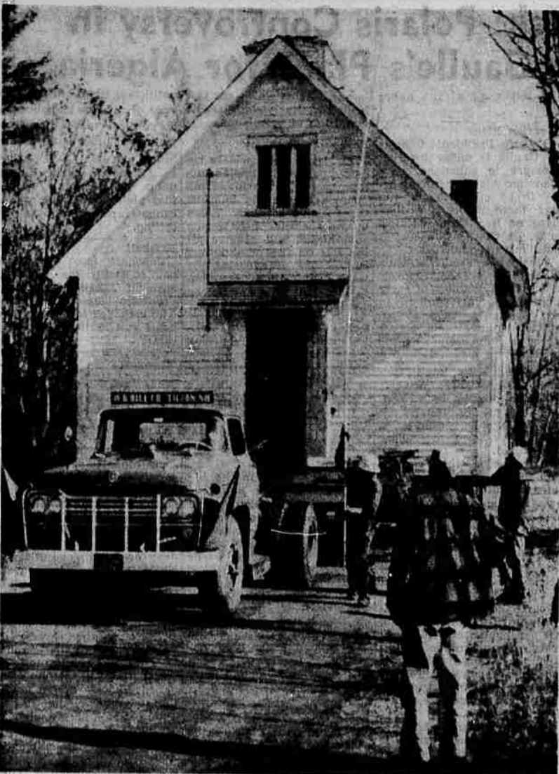
CHURCH MOVED — The Episcopal church, Chapel of the Holy Cross, built in 1893 in the town of East Weare, N. H., was moved five miles to its new location in Weare, N. H. The photo shows the church en route being guided under telephone and electric wires in North Weare. The church was relocated as the town of East Weare was evacuated to make room for a flood control project. (UPI Telephoto)
