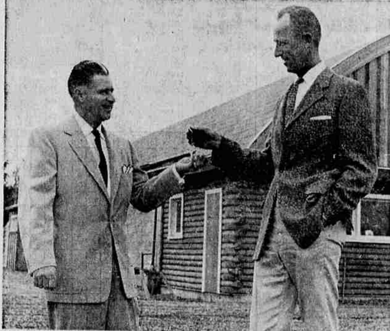
RINK READY —Rogue valley's new skating rink, the Jackson County Rollarena, located about 2½ miles south of Medford on highway 99, will be open to the public some time this coming week, according to manager Merle VanHoesen. The picture above shows VanHoesen, (left) receiving the keys to the building from Contractor Meyers Jones, an associate of Siskiyou Development corp., upon completion of the structure last week. The skating area, covered with pean veneer, will be the largest in southern Oregon, VanHoesen said. Coffee, soft drinks and sandwiches will be available at the snack bar and live music for skating will be furnished every evening except Sunday, by Jerry Miller at the organ. On Sundays the music will be taped, VanHoesen said.
