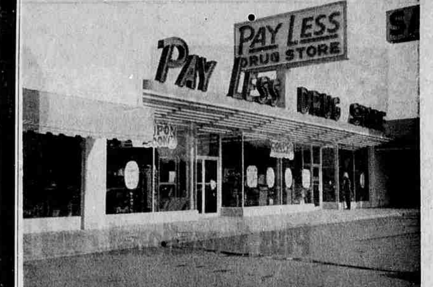
ADDITIONS—New additions to the front of the tinted glass was done by a local firm. Pay Less Drug store is the large neon sign. It not only cuts down the fading problem, on top of the building and the tinted glass, but it also removes the glare from the sun.
