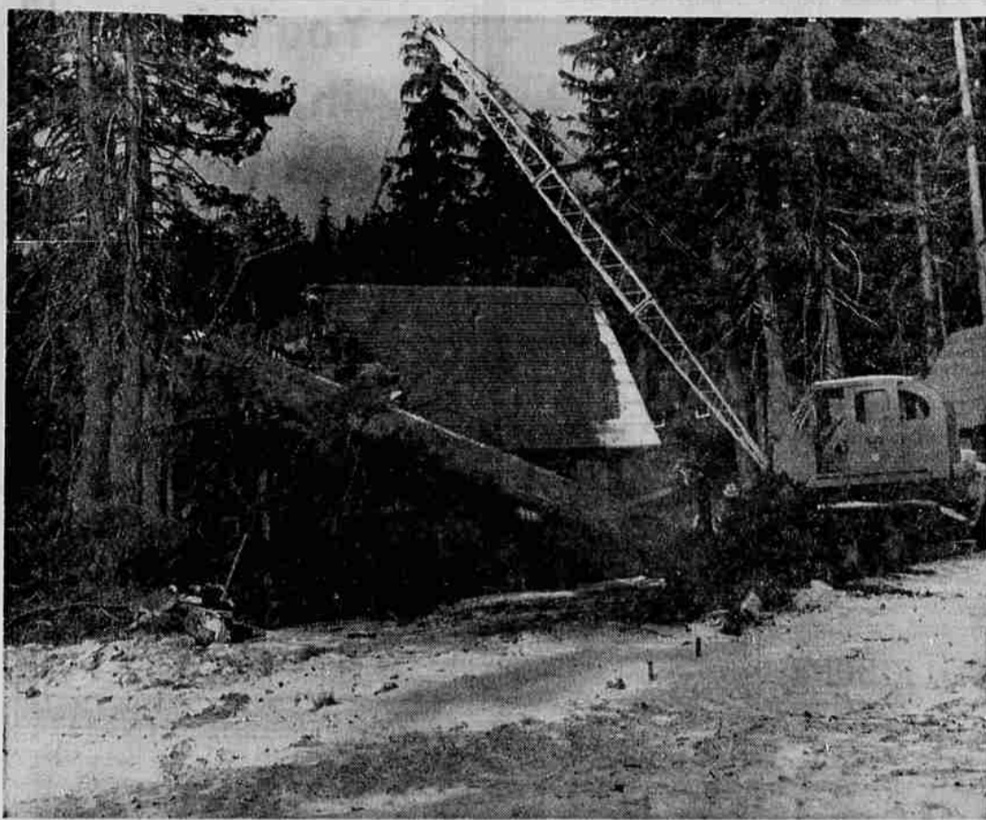
DAMAGED HOME—Workmen at Crater Lake National Park start removing a tree which was blown across the home of Mr. and Mrs. Fred Carlisle about 7:30 p.m. Sunday. The house was extensively damaged, but the Carlises escaped without injury. After the tree damaged the home, the Carlises and other residents of the park took refuge in the maintenance building until the storm subsided about 3 1/2 hours later.
