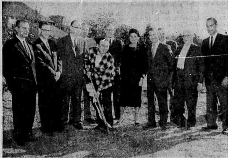
GROUND BREAKING — Arnold Bauder, (with shovel) retiring Ashland hospital board member, turned the first shovelful of dirt at the Ashland General hospital site, corner of Maple and Chestnut sts. this morning during ceremonies at 9 o'clock. Bauder was instrumental in forming plans for the $375,000 hospital. About 100 persons witnessed the event. F. R. Fairweather, Medford, is contractor for the 34-bed hospital, which is to be completed within 270 working days.
