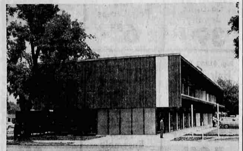
ALL WOOD CONSTRUCTION — Nearing completion on East Main st., Medford, is the Standard Insurance company building above. The structure, which will house professional offices on a rental basis, is constructed of wood with the exception of a fire-proof stairway in the center of the rear of the building. The building is expected to be in use before the end of the year.
