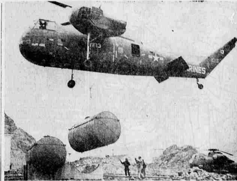
OIL TANK REPLACED —A Marine Corps helicopter eases a 7,000-pound fuel tank into a cradle at the Coast Guard lighthouse station at Farallon Island, Calif., 25 miles offshore from San Francisco, completing a unique Navy-Marine Corps-Coast Guard operation. The operation to replace the sta-
