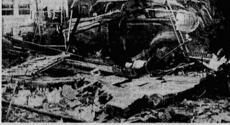
THREE ESCAPE INJURY —Three elderly women, one of them blind, escaped without injury when a gas explosion damaged their home at Beaverton. Force of the blast was enough to blow out windows of a church school a block away. The explosion was thought to have been caused by an accumulation of gas in the attic over the garage. (UPI Telephoto)
