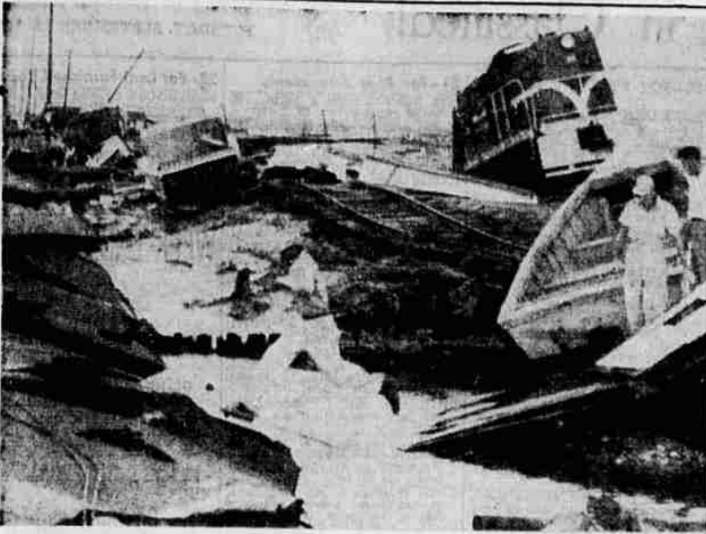
HURRICANE DAMAGE —A clean-up worker jumps across a flooded ditch on a causeway between Morehead and Beaufort, N.C. A section of the road and railway were torn up, boats were blown or washed up from an inlet 100 yards to the left. The switch engine was on the track when a small bridge fell. This area was one of the hardest hit by hurricane Donna. (UPI Telephoto)
