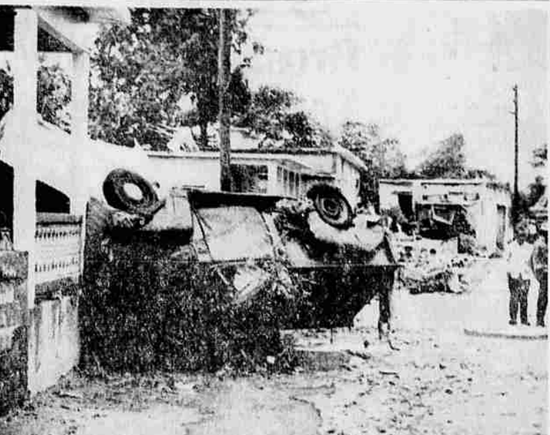
HURRICANE DAMAGE — This was the scene in Puerto Rico after winds of Hurricane Donna lashed the area earlier in the week. People walk past an upended vehicle that slammed into the side of a house during the storm. Shortage of water raised a typhus threat and an emergency mass inoculation program is under way. (UPI Telephoto)
