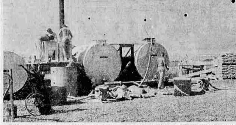
MIXING BORATE —Crews are shown above mixing borate "slurry" at the Medford airport. The slurry is pumped from a small mixing tank to two 2,000-gallon storage tanks. New equipment which is expected soon will include a larger mixer, another borate storage tank, and a water storage tank.
