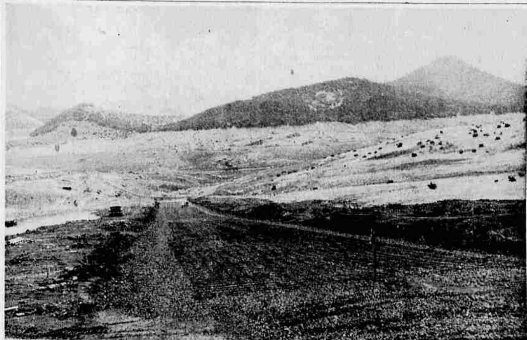
NEW BOAT RAMP —Construction is expected to be completed by Sept. 30 on the concrete boat ramp at Emigrant lake. The boat ramp, under contract by the bureau of reclamation, is part of the work being done in the Talent irrigation district. Following the laying of steel matting on the gravel a concrete strip 20 by 625 feet will be poured. BR officials reported that the length was needed to accommodate boats as the water level of the lake will fluctuate.
