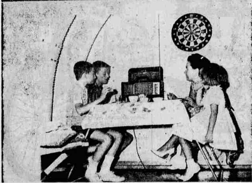
UNDERGROUND SHELTER —Combo showing the family underground shelter for fallout protection was unveiled in Chicago Tuesday by Gov. Leo A. Heeg, director of the office of civil defense mobilization. Installation of the "backyard shelter" varies, depending on construction conditions, at a cost of $1,195. A waterproofing asphalt material is applied and the entire shelter is then wrapped with a polyethylene sheet. Installation time is two or three working days. (UPI Telephoto)
