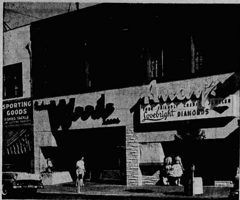
NEW STORE FRONT —Two modern store fronts have taken the place of the old M and M Department store on Main st. in Medford. The new fronts, belonging to Andy's and Parker Woods Leons, are of stone and an interesting optical tile. The tiles are so laid that they give the effect of three dimensional blocks. Parker Woods Leons, which opened Thursday, also has an entrance facing toward the Park and Shop lot in the rear.
