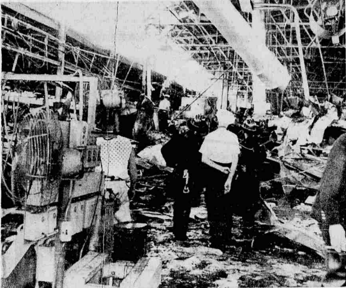
EXPLOSION LIFTS ROOF—Part of the roof of the Rheem Manufacturing Co. at Houston, Tex., was blown off in a violent explosion of a lacquer oven Monday. Firemen are shown extinguishing a flash fire that occurred after the blast. Four persons were reported killed. (UPI Telephoto)
