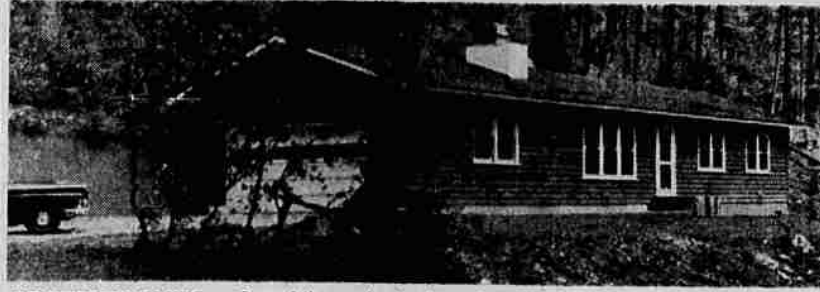
AT OREGON CAVES — One of the projects under Mission 66 at Oregon Caves is this new residence for the management assistant there. The building was completed this spring and will be used by the only permanent park service employee in this area, according to Otto M. Brown, park superintendent. Along with new parking areas, picnicking space, and orientation facilities, this project will prepare the monument for an anticipated 100,000 visitors per year in 1966, completion date for the National Park service's development program. (NPS Photo)
