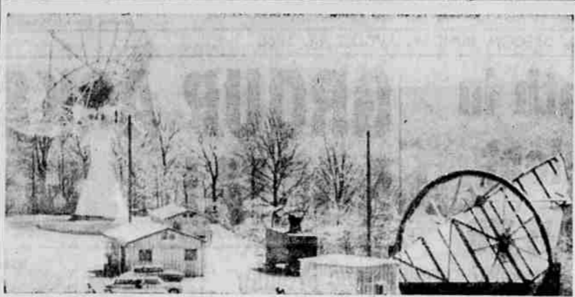
TERMINAL TO SPACE - This is the Bell Telephone Laboratories "telephone terminal to outer space" at Crawford Hill in Holmdel, N. J. Signals were bounced from here, via Echo I communications satellite, to the Jet Propulsion Laboratory in Goldstone, Calif. In foreground at right is the unique "horn-reflector" antenna used as a receiver for the satellite communication system. The transmitter, a 60-foot "dish," is at top left. (UPI Telephoto)
