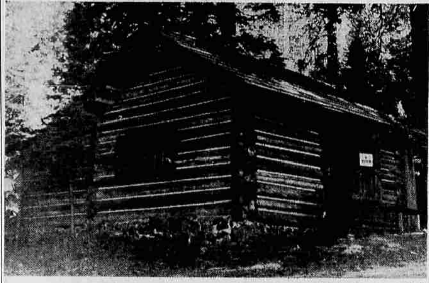
CARETAKERS CABIN —This large comfortable looking cabin is being used by the caretaker and concession operator at Howard Prairie reservoir. For the general public, Bob Johnston, of Johnston stores, Medford, hopes to have house trailers located north of the picnic grounds.
