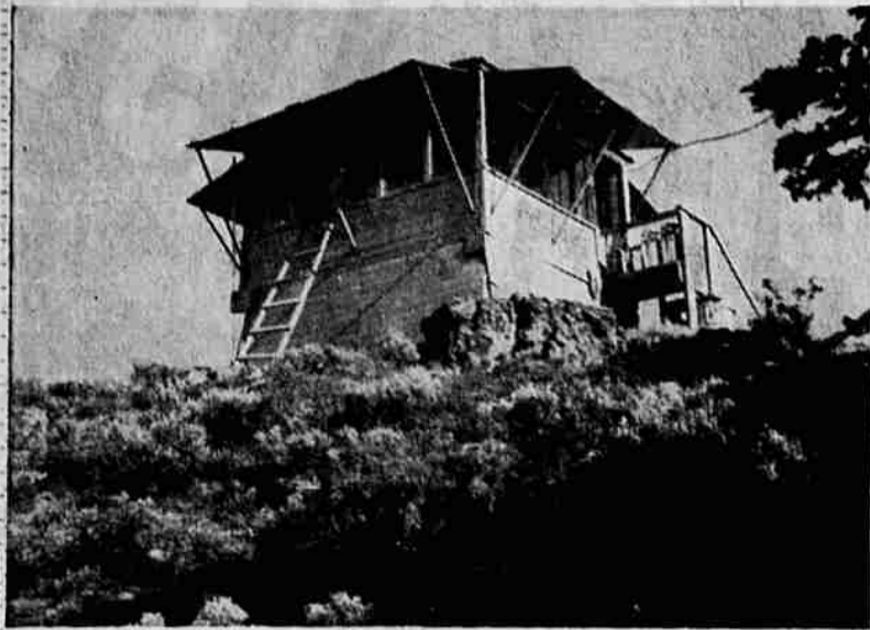
HALF-STORY —Soda mountain lookout is a half-story structure located on the Greensprings mountain east of Ashland. Shutters on the building help reduce the glare of the sun and assist the lookout in spotting small fires.
