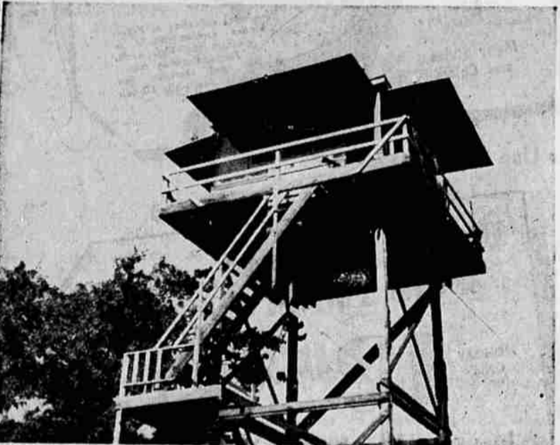
BURNT PEAK TOWER —The Burnt peak tower is 29 feet high with two flights of stairs leading to the top. Safety on lookouts is stressed both during training sessions and on the job to help prevent accidents resulting from falls.
