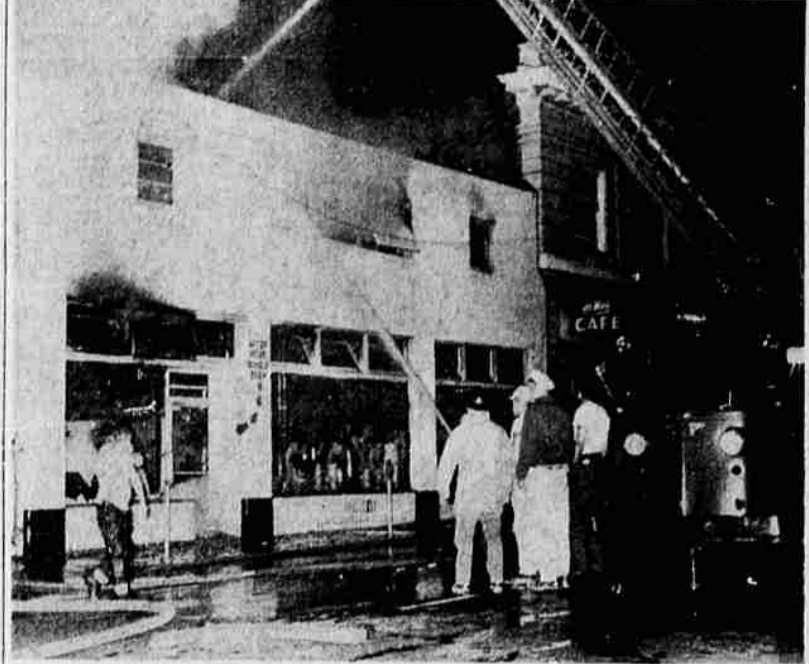
GENERAL ALARM —Shown in initial operations is one crew of the Medford fire department who turned out for a "general alarm" fire this morning at Dumas Domestic Laundry and Dry Cleaners, 30 North Riverside ave. Damage was estimated $150,000 to $200,000. The dry cleaning areas plus most office records were saved.
