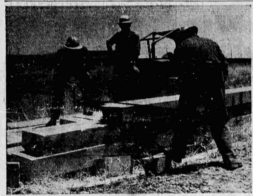
MILL SITE—Preliminary work for the construction of the new Medford Corporation plywood mill at the north end of town included the building of a bridge over an irrigation ditch so heavy machinery could cross. To cut the heavy timbers for the bridge, a crew of men, above, made use of an "old-fashioned" cross cut saw. The mill, when completed, will employ some 200 men with a payroll in excess of $1 million, and could be expanded to employ 300 in the future, according to Medford Corporation directors. By next week, construction of the plant should be in full swing, a spokesman said.
