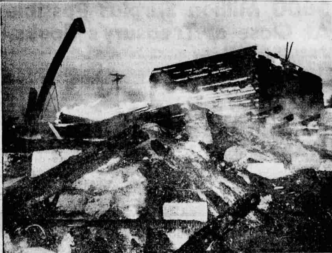
ONLY RUBBLE REMAINS —Only smoking ruins remained after a fire swept through the tiny town of Monitor, Ore., southeast of Woodburn, late Wednesday. The fire caused an estimated $70,000 damage before being quenched by firemen and scores of volunteers. (UPI Telephoto)
