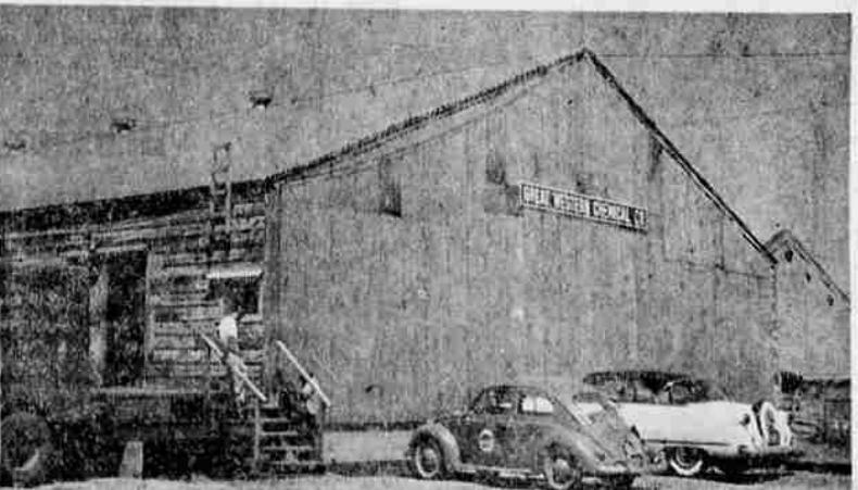
CHEMICAL OUTLET — Among the more recent additions to the White City industrial area businesses is the distribution center for the Great West Chemical company, shown above. The company furnishes chemicals used in sealing and finishing plywood.
