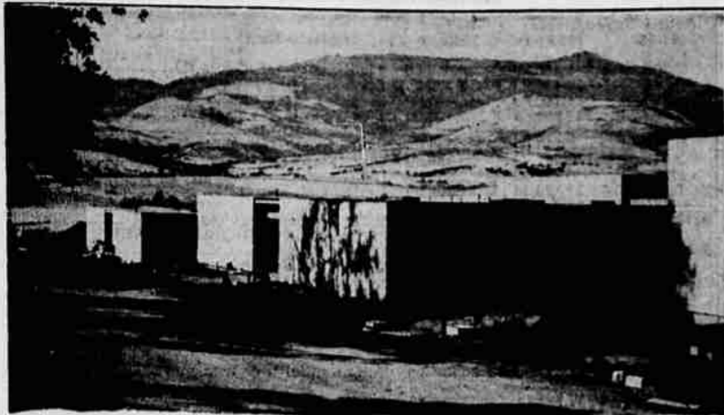
AHEAD OF SCHEDULE —Work on Ashland's new junior high school on Walker ave. is 75 per cent complete and Contractors Graff and James of Medford report they are ahead of schedule. Construction began last December and completion deadline is Sept. 1. School Superintendent Stanley Jobe expects an enrollment of nearly 700 seventh, eighth and ninth graders this fall.
