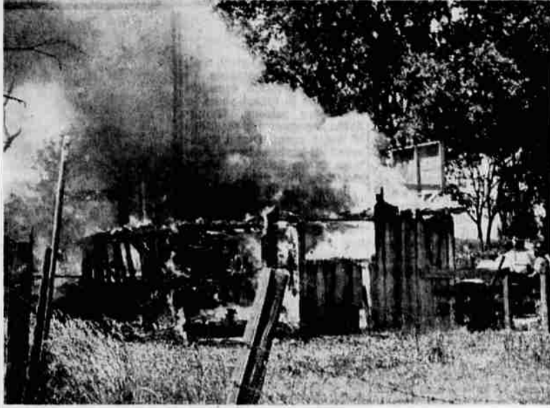
FIRE DESTROYS SHED—Fire which broke out about noon Friday completely destroyed a three-unit structure behind a residence at 871 Cherry st. The old structure, consisting of three joined sections, a records office,
