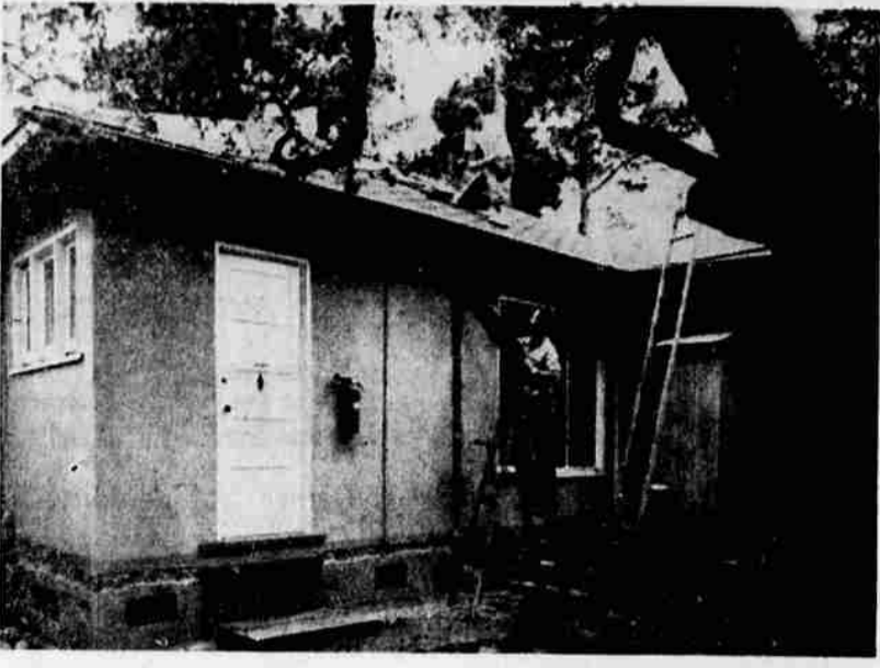
HOUSE MOVED, TREES STAY — In the forested town of Carmel, Calif., where trees are sacrosanct, a city councilman made a Solomon-like decision on how to remove the Arthur F. White home from a lot recently acquired by the town, without cutting down pines and oaks in the way — just by sawing the building in half. Workmen started to cut the residence in two parts, so that each may be eased through the woods and rejoined at a new location across the street. (UPI Telephoto)
