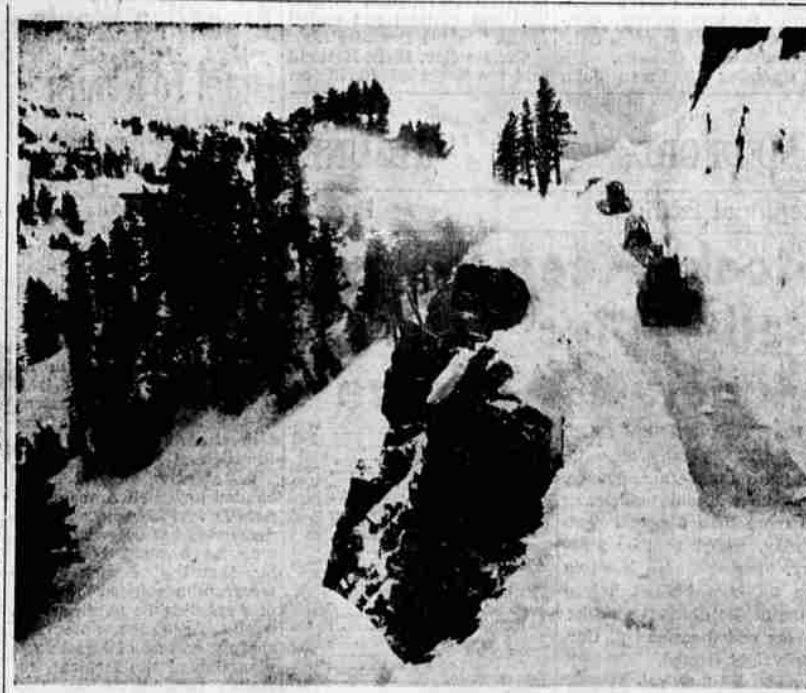
CLEARING ENTRANCE—Bulldozers and rotary snow plow are shown above clearing the rim road at Crater Lake National park so the north entrance road may be open by June 15. Heavy snowfall in April and May handicapped park crews in their efforts to clear the winter's snow from roads and
