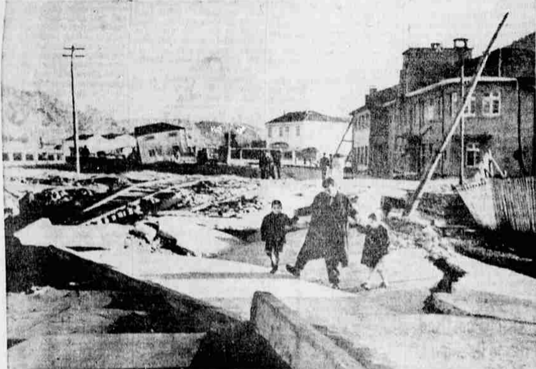
QUAKE DEVASTATION - Residents of Puerto Montt, Chile, walk along a bent and broken sidewalk after violent earthquakes devastated the area. Two new quakes have been reported in the area and seismologists say the second
