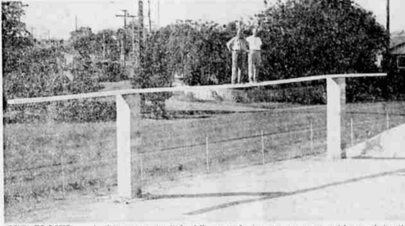
ODD PLANK — A thin concrete "plank" some 60 feet long, that bends like spring steel, is currently on display at Builder's Supply company, 727 West McAndrews rd., Medford. It is made of pre-stressed concrete. Pre-stressed concrete beams and wall panels are now being manufactured by the Medford firm on a special pre-stressing bed recently installed. Tension of thousands of pounds is put on steel cable used in the forms and is released after the concrete has set, giving the material its unusual strength. Standing on the plank, which is only 3 1/2 inches thick, above, is Plant Owner M. R. Gibbons and Employee Max Hawks. There are only three other pre-stressing plants in the state of Oregon.
